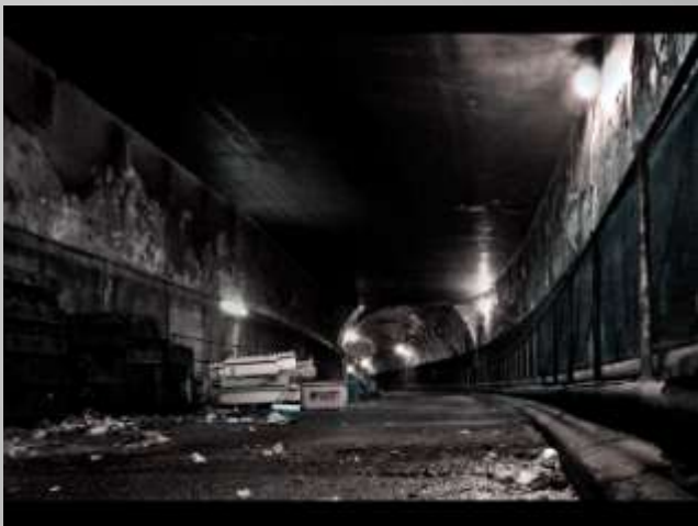
Old Mersey Tunnel (Stuart Worrall)
